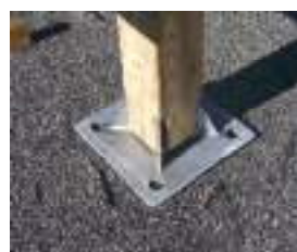
Platine 400x400Ep 10 mm
